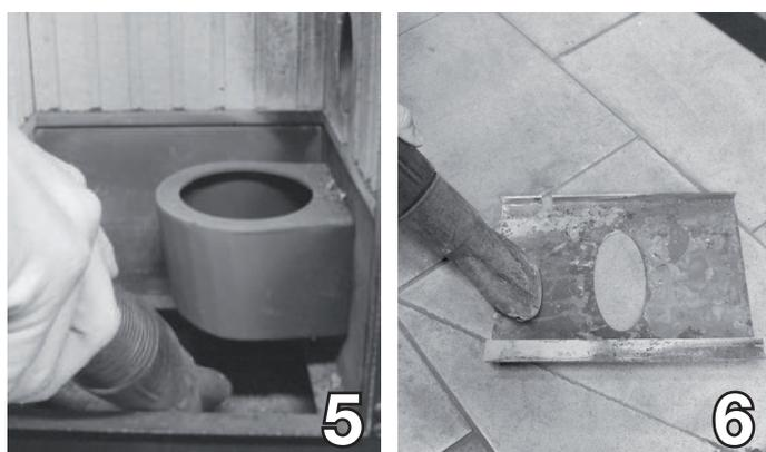
Remove the combustion chamber floor with the aid of a screwdriver and with a vacuum cleaner, clean under the plate. (foto 5)
