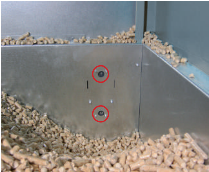
Sensor level of fuel in the tank
