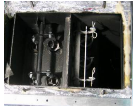
Device for automatic cleaning of the pipes for the passage of fumes
