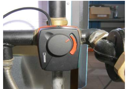
4-way mixing valve for perfect protection from return flows
